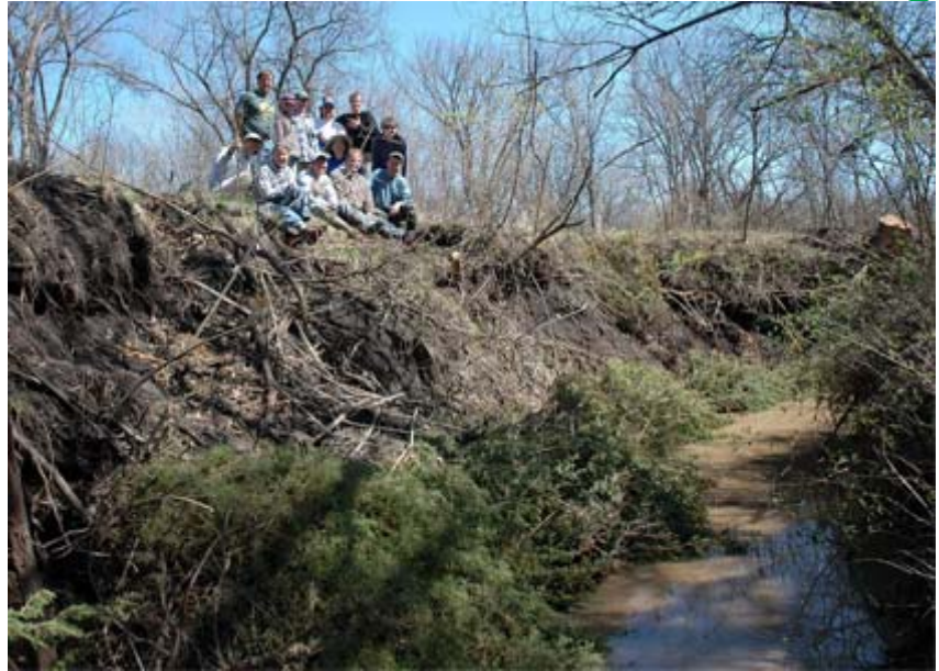
This photo shows the cedar trees just after they were anchored into the streambank in April, and 12 of the 20 volunteers who completed the revetment: sitting from left: Jill Baringer, Durand Reiber, Katie Speicher, Mary Beth Petr, Will Boyer & Bill Wood. Back from left: Cosmo Canacari, Genevieve Voight, Joanna Voight, Ryan Chapman, Colby Pearson, and Karen Warner. Charlie Barden from KSU Research and Extension took the photo. Other volunteers were Alison Reber, Cindy Riling, Jeff and Cris Bandle, Jill Giele, Paige Blair and Melanie Bird.
