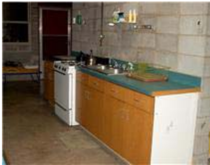
New cabinets in Arkalooka's kitchen.
