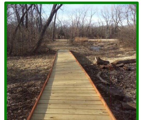
Enjoy the recently completed Sherwood Bridge on Trails Day! Gwen Macpherson led the work to build the long bridge, sometimes with student help. The bridge spans 35 feet, plus 15' ramps on both ends! Thank you Gwen!
